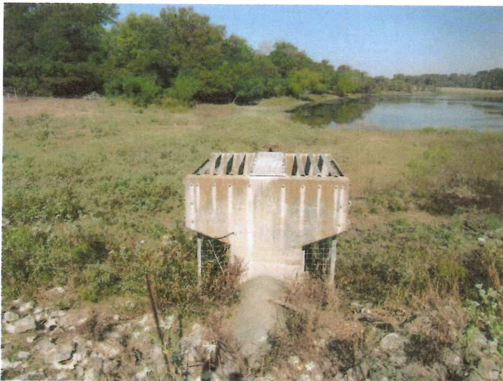
Photograph 8: Principal Spillway inlet and reservoir.
