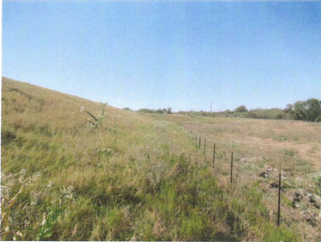
Photograph 3: Upstream looking right.
