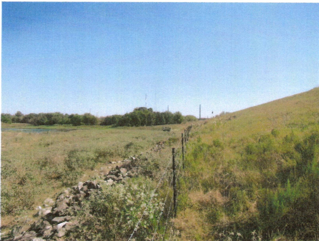
Photograph 4: Upstream looking left. Note vegetation among riprap.
