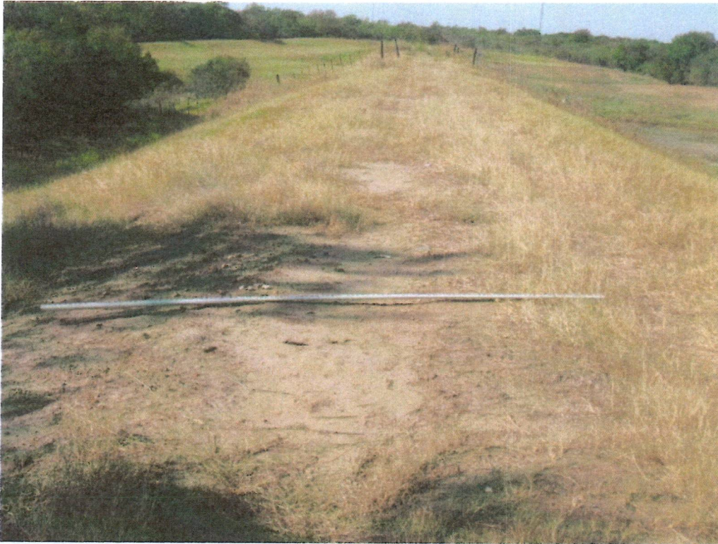
Photograph 1. Crest looking right. Note bare spots.
