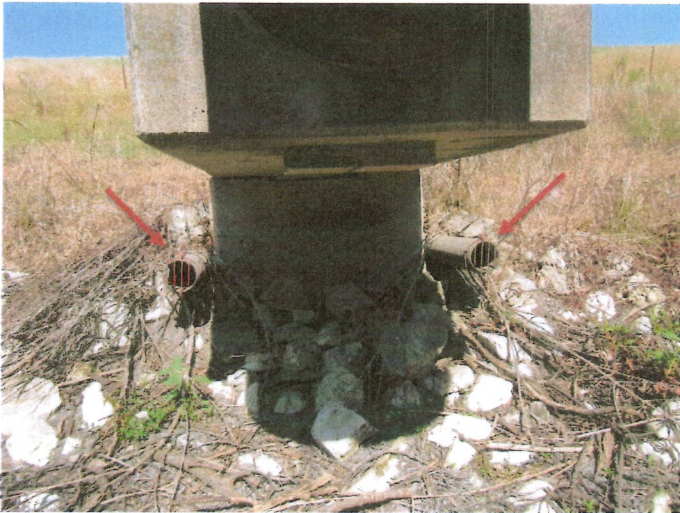
Photograph 12: Toe drain outlets.
