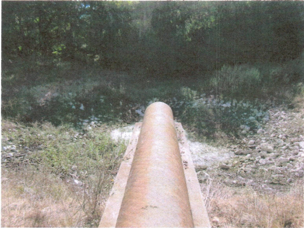
Photograph 9: Principal Spillway outlet pipe and plunge pool.
