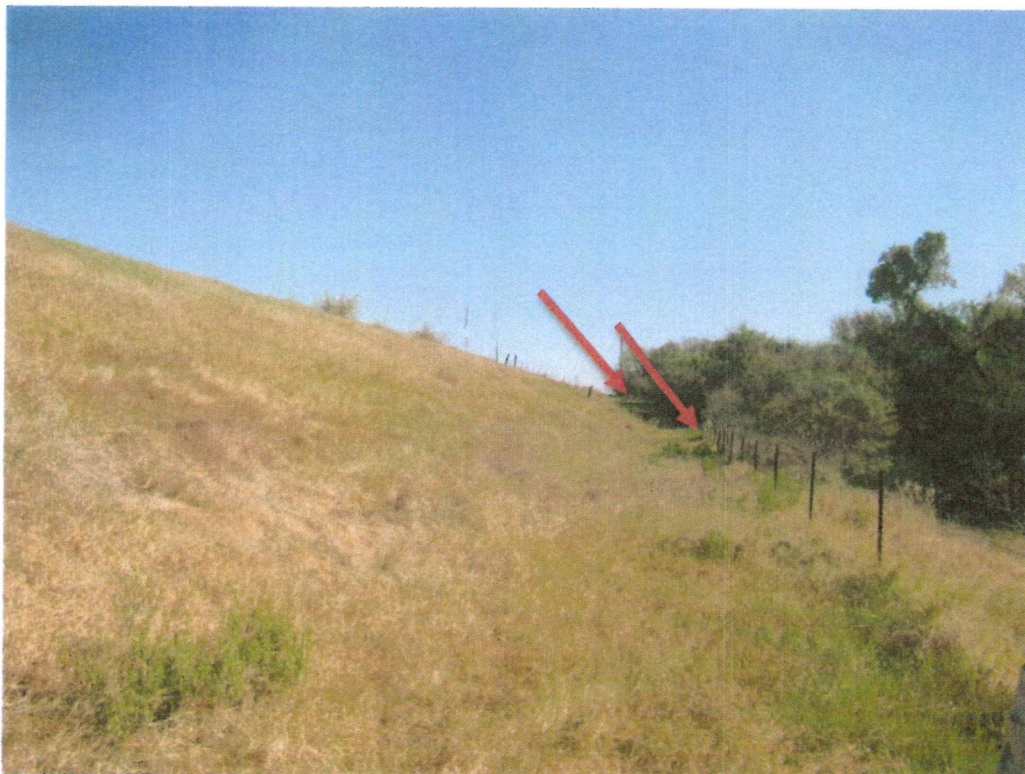
Photograph 6: Downstream slope looking left. Note brush new toe area.
