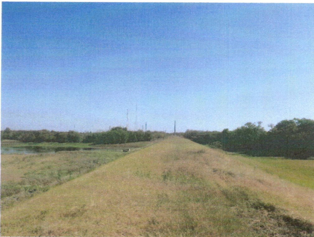
Photograph 2. Crest looking left.
