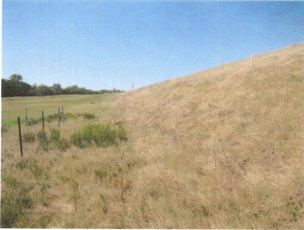
Photograph 7: Downstream slope looking right.
