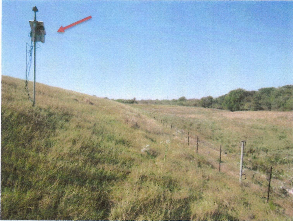
Photograph 15: Out of service weather station.
